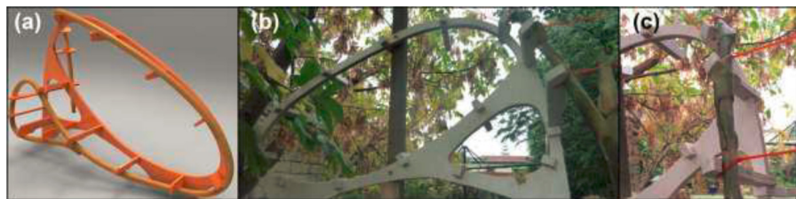
Figure 5. Bamboo shape modification over substructures (Vittouris, 2011)
